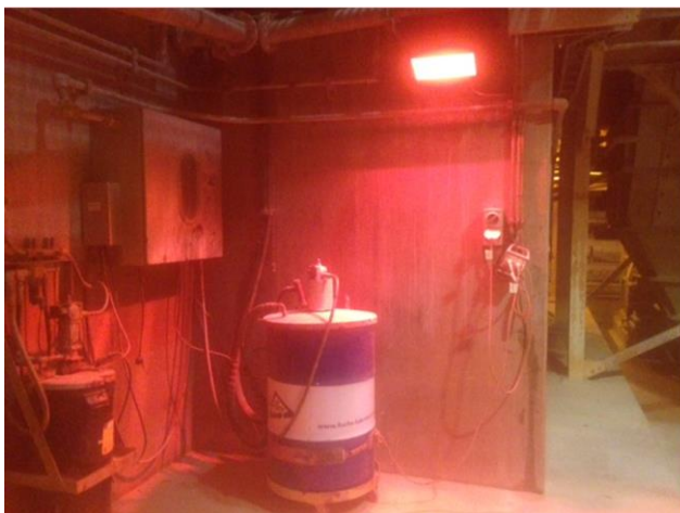
An infrared heater projects heat from a distance so can be mounted on a nearby wall or ceiling.
